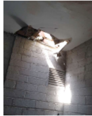
The Willows: Examples of defects Top: ceiling damaged by roofer Visible gap in chimney flashing Vent pipe replaced where penetrating roof but existing hole not repaired Centre: poor workmanship: sundry leaks, incomplete lining to roof Bottom: leaking replacement downpipes, possibly undersized, and displaced leak guard Unfixed and poorly installed soffit
